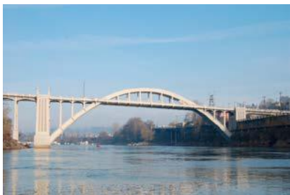
New Oregon City Arch Bridge
